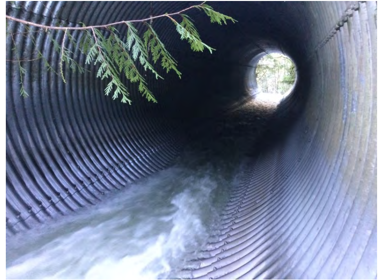
Looking through from inlet
